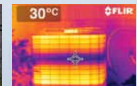
What a thermal imaging camera sees.
