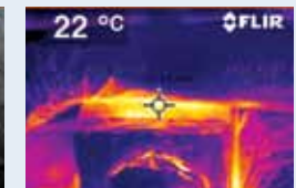
What a thermal imaging camera sees.
